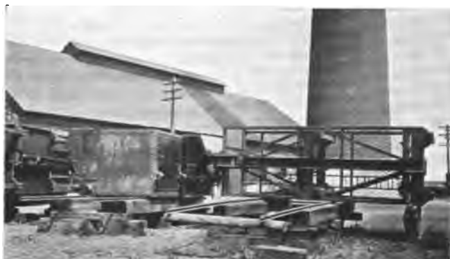
B. SKIPS AND MAN CAR AT RED JACKET VERTICAL SHAFT.
